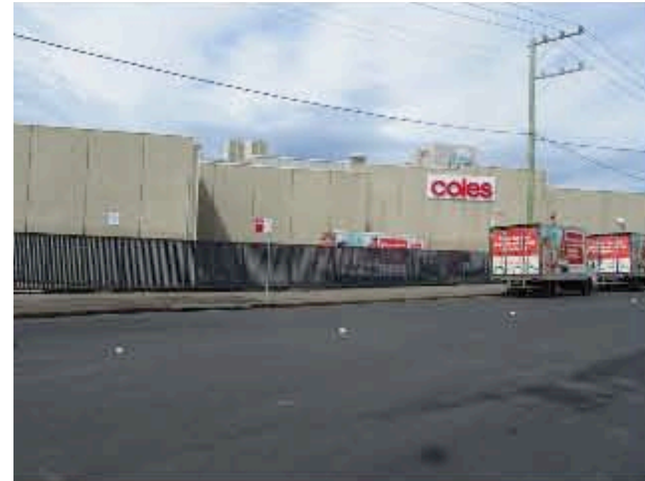
08. Sharp Street facing East Coles loading dock
