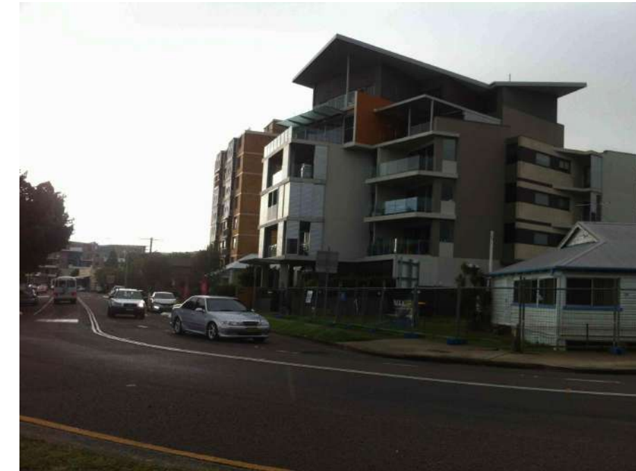
10. Brooks Parade facing North Deck Apartments in foreground
